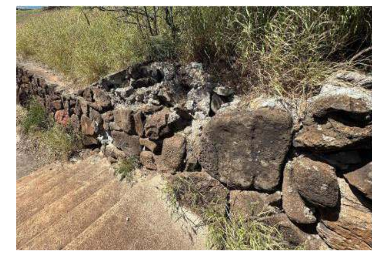
4 ROCK WALL REPAIR
